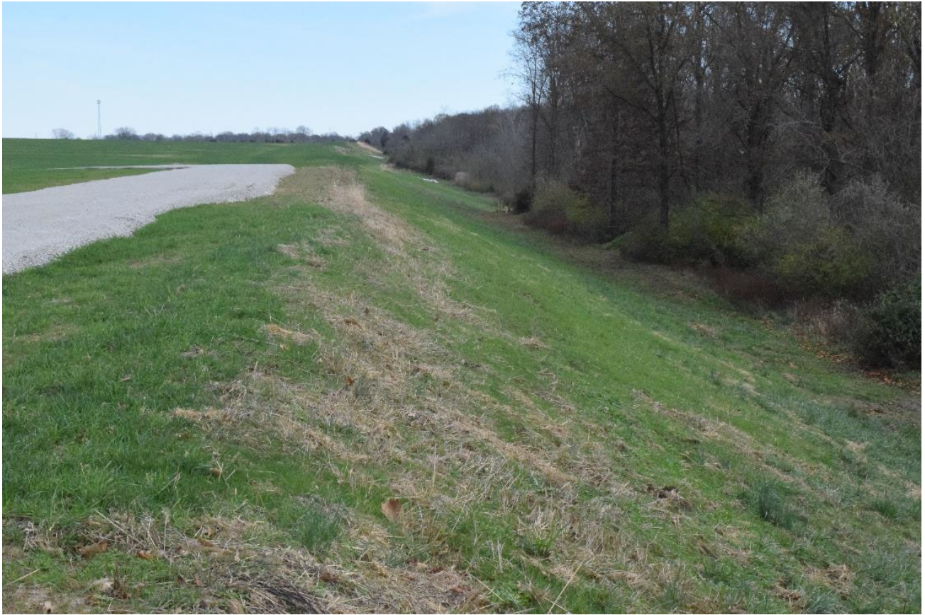
Closed ash pond – south side
