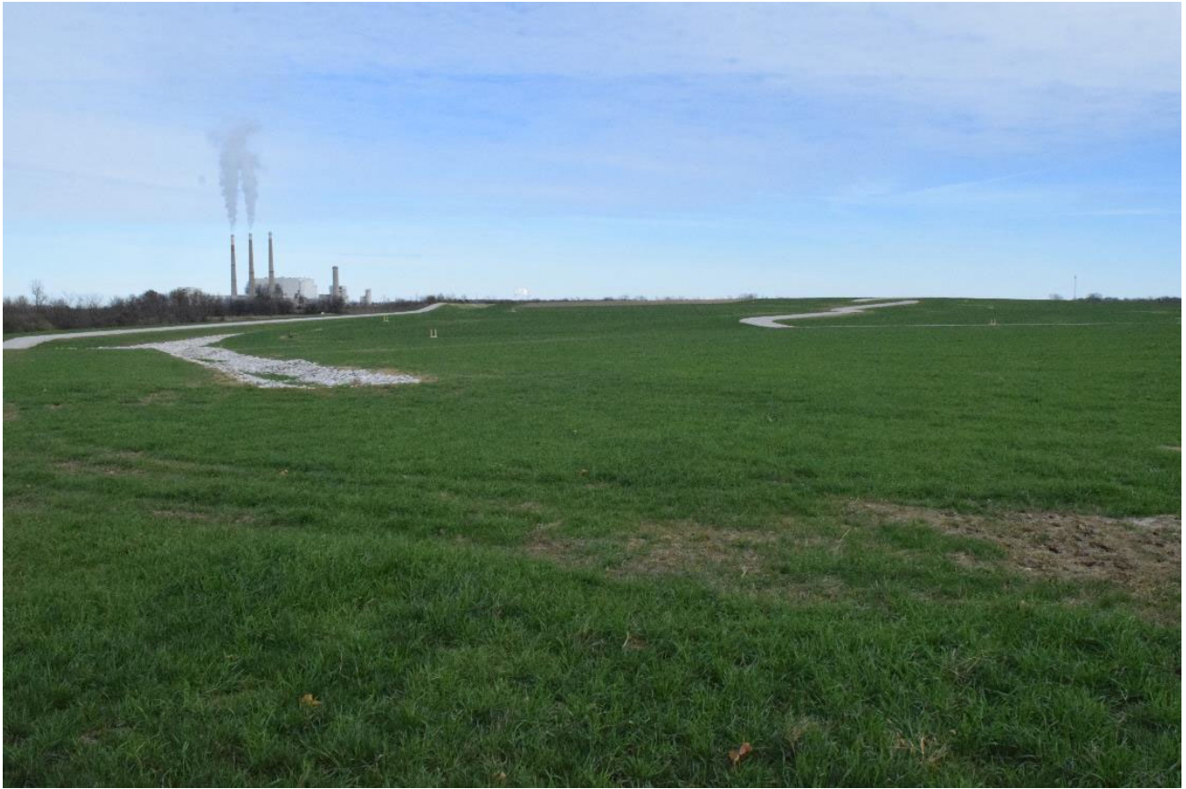
Closed ash pond – interior
