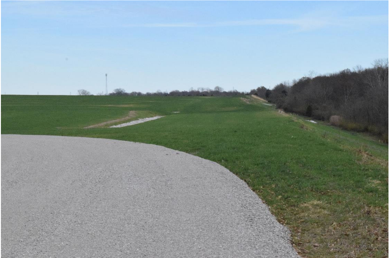
Closed ash pond – interior
